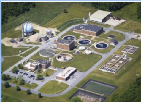
Figure 2. Derry Township Municipal Authority's Clearwater Road WWTP, Hershey, PA.
